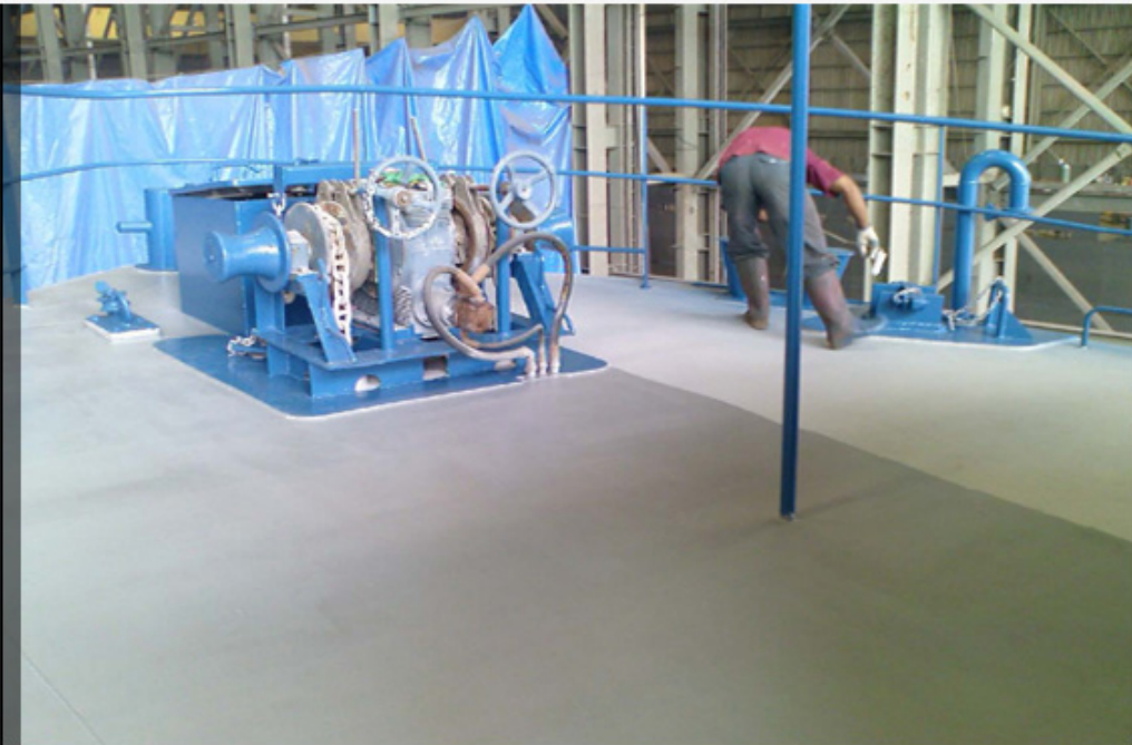
Anchor winch and forward deck.
